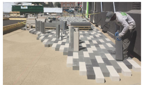
Figure 6. Installing planks on uncompacted bedding sand.
