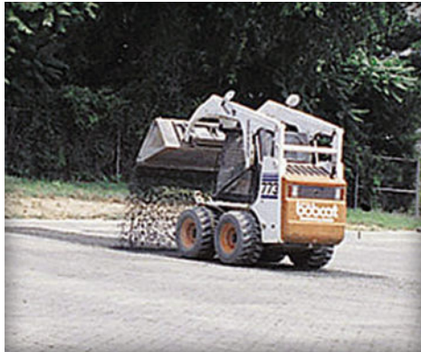
Figure 28. Various methods of filling and sweeping PICP joints.
