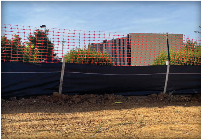
Figure 10. Typical silt fence application.
