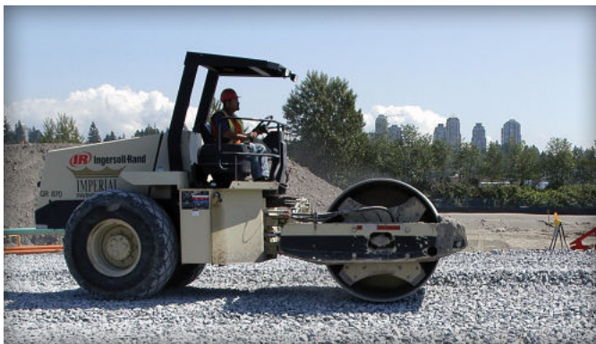
Figure 15. A 10 ton (9 T) vibratory roller compactor settles ASTM No. 2 stone subbase for a large shopping center parking lot.
